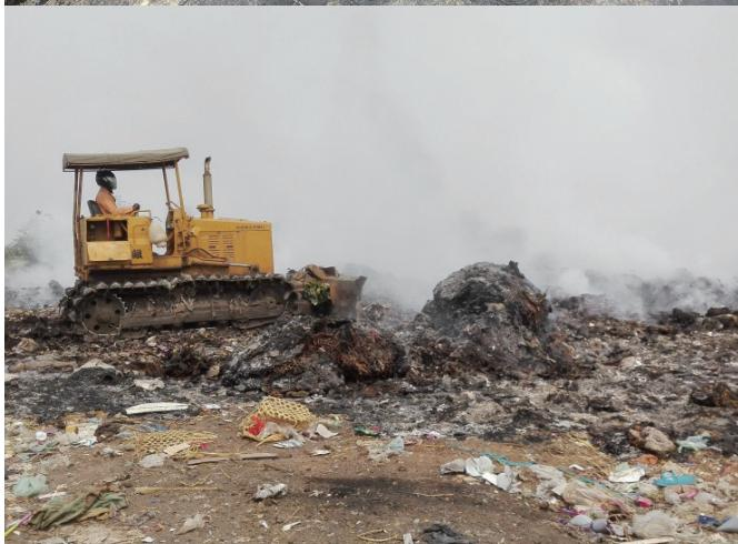
Figure 13: Extinguishing Landfill Fire using Water and Soil
