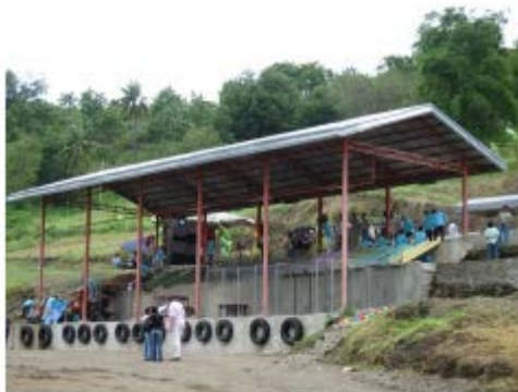
Materials Recovery Facility
