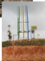
Semi Controlled Landfill
