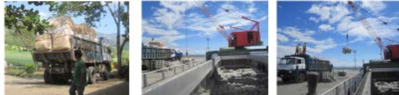
Hauling of waste materials for delivery to SCC Port
