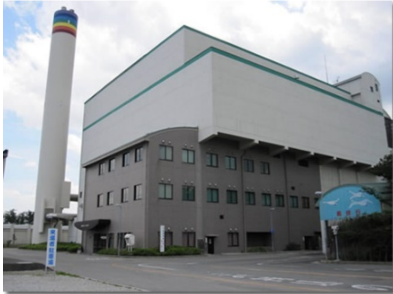
Yonago city clean center (waste-to-energy power generation)
