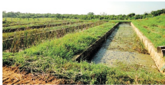
c) Treatment wetland ditches installed in a semi-engineered landfill in Addalatchenei, Sri Lanka
