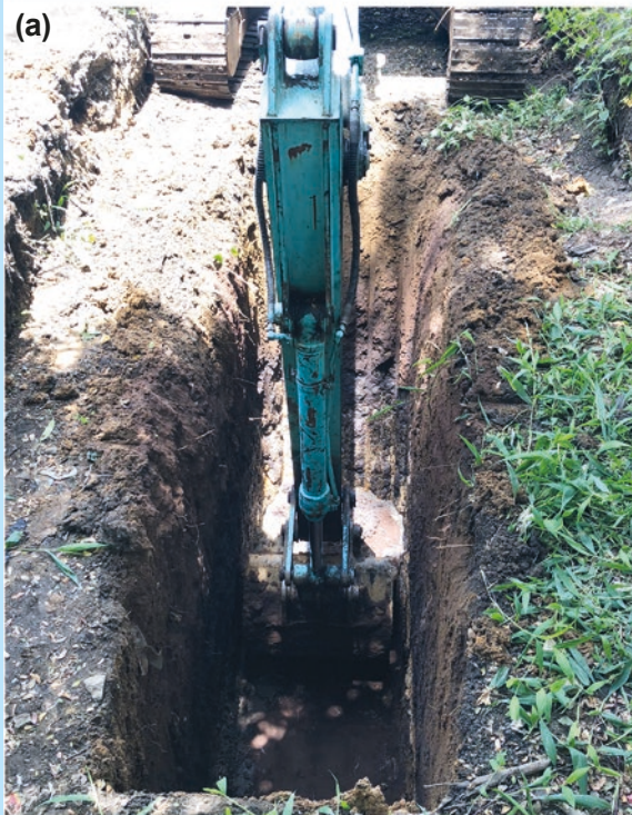
a) Trench excavation across the groundwater flow paths to install PRB materials (1 m wide, 5 m deep and 60 m long) at Sundarapola dumpsite, Kurunegala, Sri Lanka
