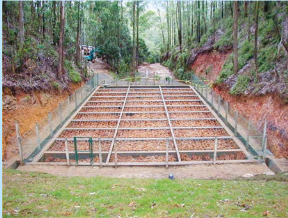
a) Attached growth biofilm (Coconut fiber Biofilm - COTS) treatment system installed at the Moonplains rehabilitated dumpsite in Nuwara Eliya, Sri Lanka
