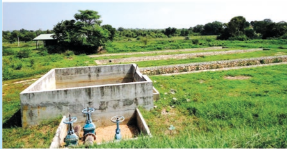
c) Series of stabilization ponds installed in a semi-engineered landfill in Ampare, Sri Lanka
