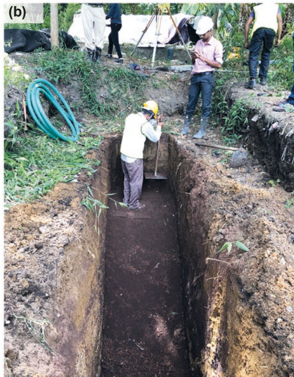
b) Trench filling by PRB materials (Biochar+ clay brick particles + dense clay) and compaction to finish the installation
