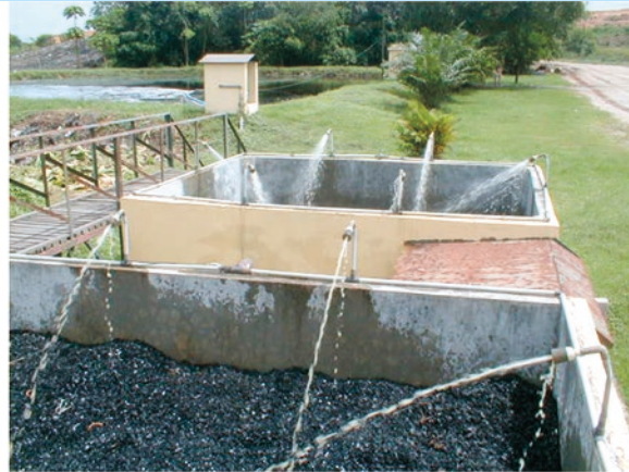
b) Attached growth biofilm on a roughing filter installed at a rehabilitated landfill in Malaysia
