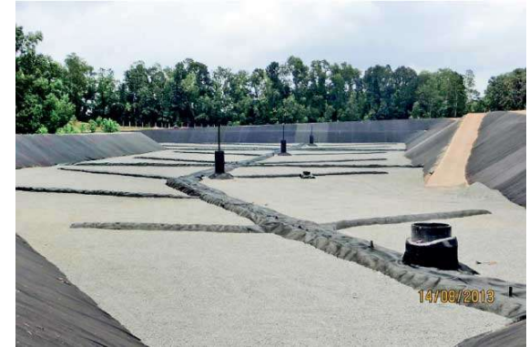
Sanitary land filling
