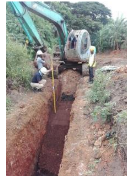
Construction of Permeable Reactive Barrier (PRB) at Sundarapola Dumpsite, Kurunegala
